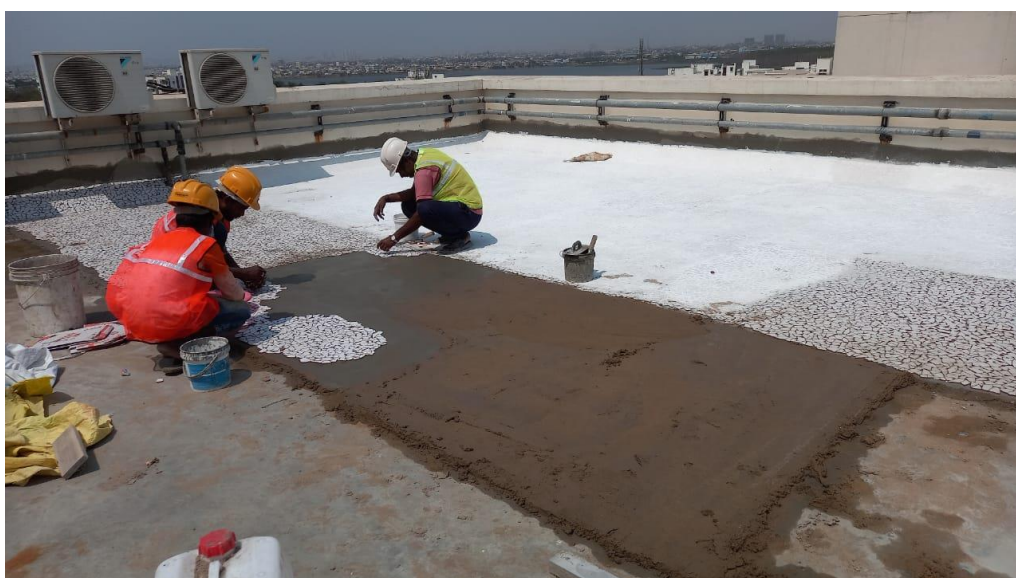
Workers build a cool roof at the premises of ASCI, Hyderabad City, Telangana.
